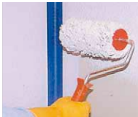
Applying Aquaflex WPU on a wall with a roller
