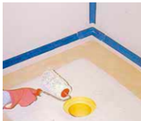
Spreading Aquaflex WPU around the drain in a shower cubicle
