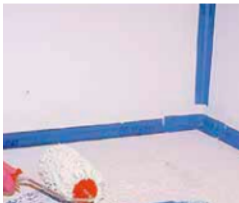
The special piece of Mapeband embedded in the Aquaflex WPU
