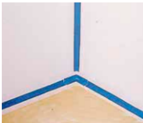
Bathroom wall waterproofed with Aquaflex WPU and Mapeband
