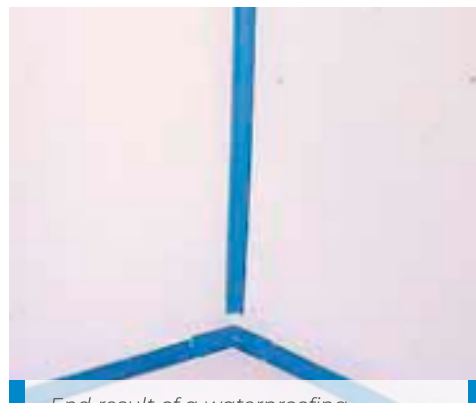
End result of a waterproofing treatment using Aquaflex WPU and Mapeband
