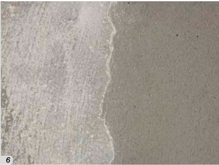
Fig. 6 - The surface of cementitious grout with efflorescence
