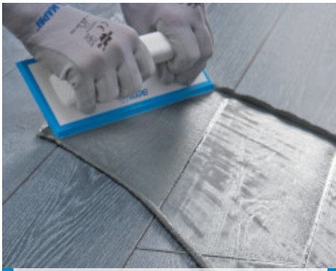
Spreading Ultracolor Plus on wood-effect porcelain floor tiles with a rubber float
