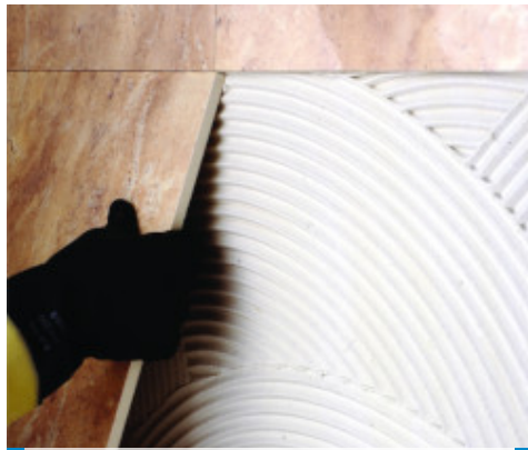
Laying large-sized porcelain tiles on walls
