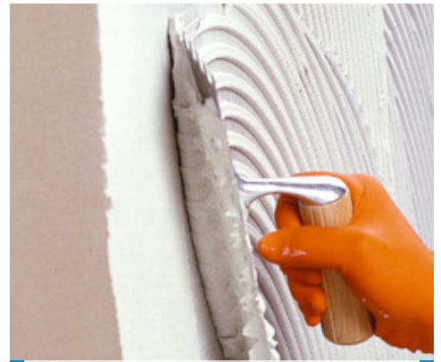
Spreading Tixobond Fine S1 on a substrate
