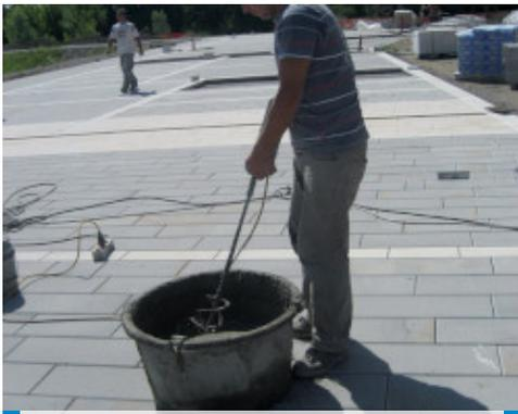
Mix Mapestone PFS 2 Visco with water only using a mixing attachment or cement mixer
